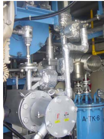
d. Chemical Addition Tanks
