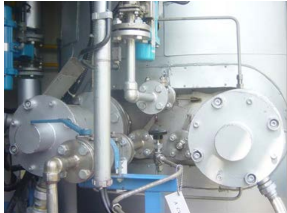
b. Reactor Face
