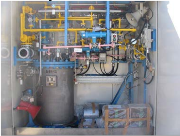
c. Sodium Dispersion Section – sodium dispersion holding and measuring tanks
