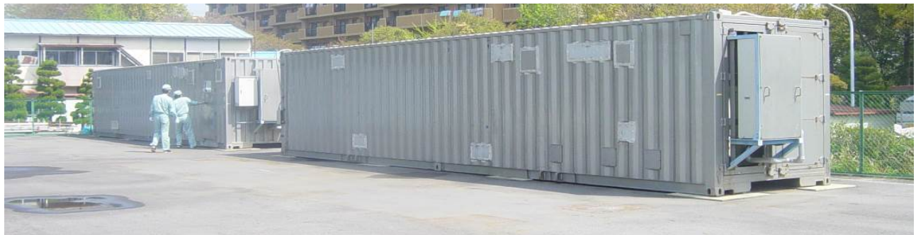
a. ISO Containers Housing MPU-3
