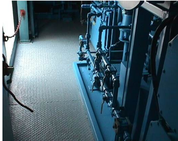
f. Built in Secondary Oil Spill Containment System
